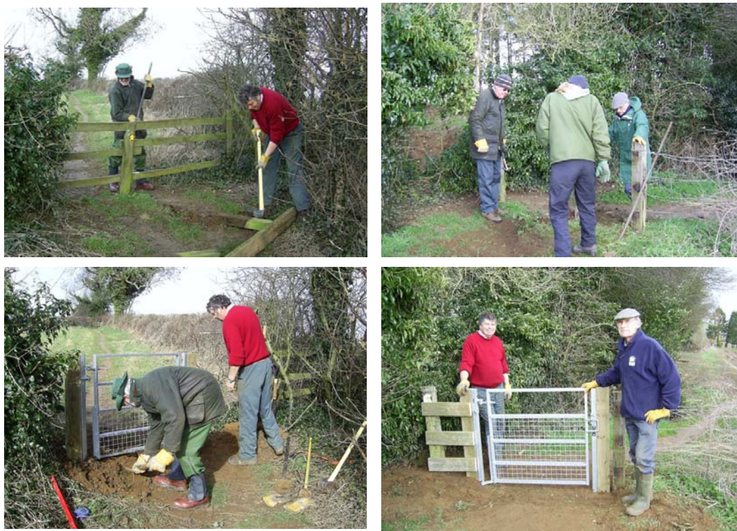
Epwell village volunteers & Cotswolds Voluntary Wardens replacing a stile with a pedestrian gate
